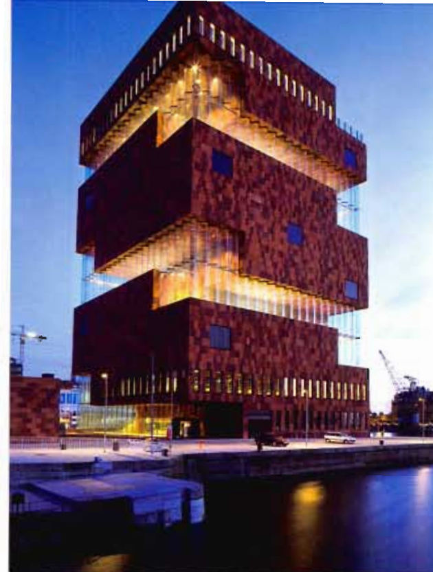
◀ Located along Antwerp's waterfront, the Museum aan de Stroom's facade features spans of up to 18 feet of corrugated glass. Photo © Sara Blee
