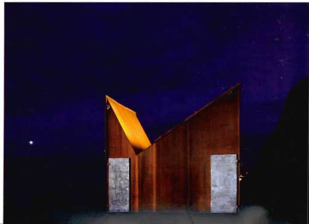
The durable construction of the 37sm bathroom facility in Akkarvikodden, Lofoten in Northern Norway replaces an earlier restroom that was swept up by the Arctic winds. Photo © Paul Warchol
