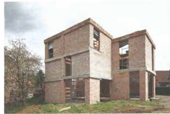
BLAF Architecten – dnA house, Asse
