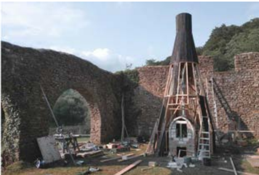
Fig.14 - The hoven being built
