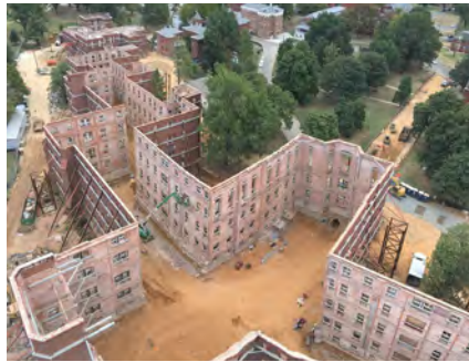
'brick for permanence and the future ruin' St-Elizabeth's Hospital renovation, Washington DC Photo unknown
