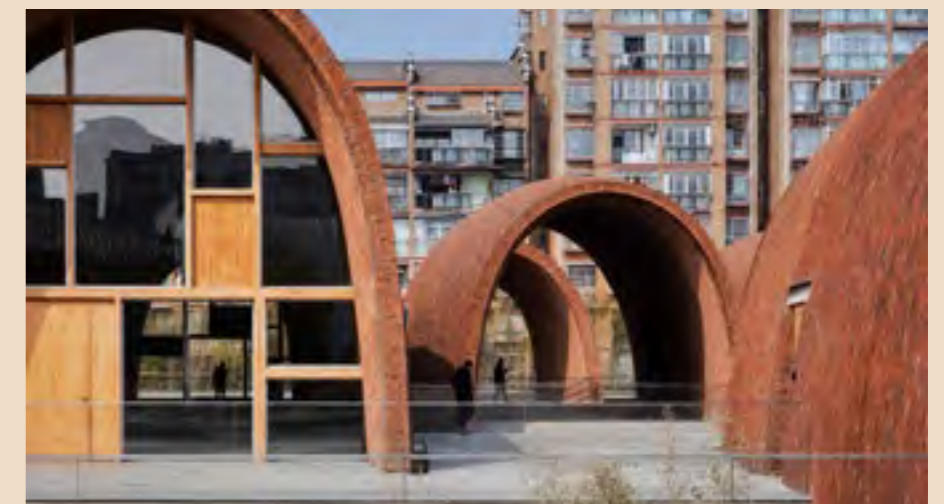
The brick vaults at Studio Zhu-Pei’s Imperial Kiln Museum, Jingdezhen, China, are based on the form of a traditional kiln.
