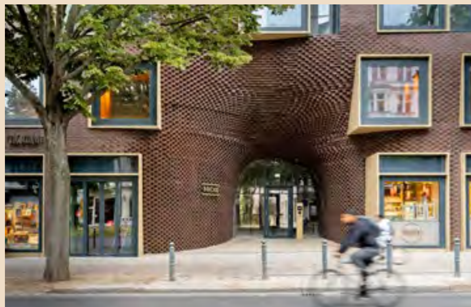
Curved brickwork is a salient feature of GRAFT architect's remodeling of a decommissioned post office in Berlin, Germany.
