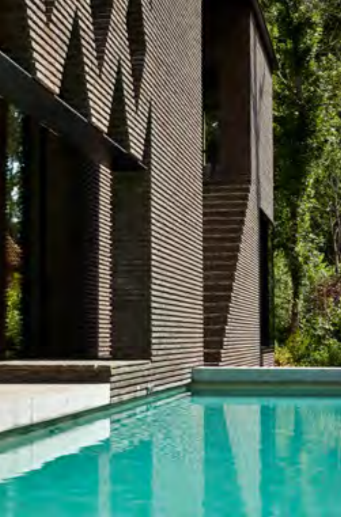
At House DG in Belgium, Lens o ass architects have created a brickwork diamond mesh to shield the interior from direct sunlight.
