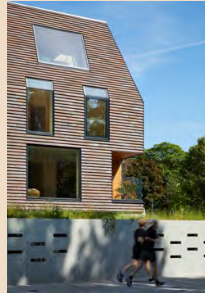
Petersen Tegl bricks are used to construct the irregular angular forms of two sister buildings at The Rye in Peckham, London.
