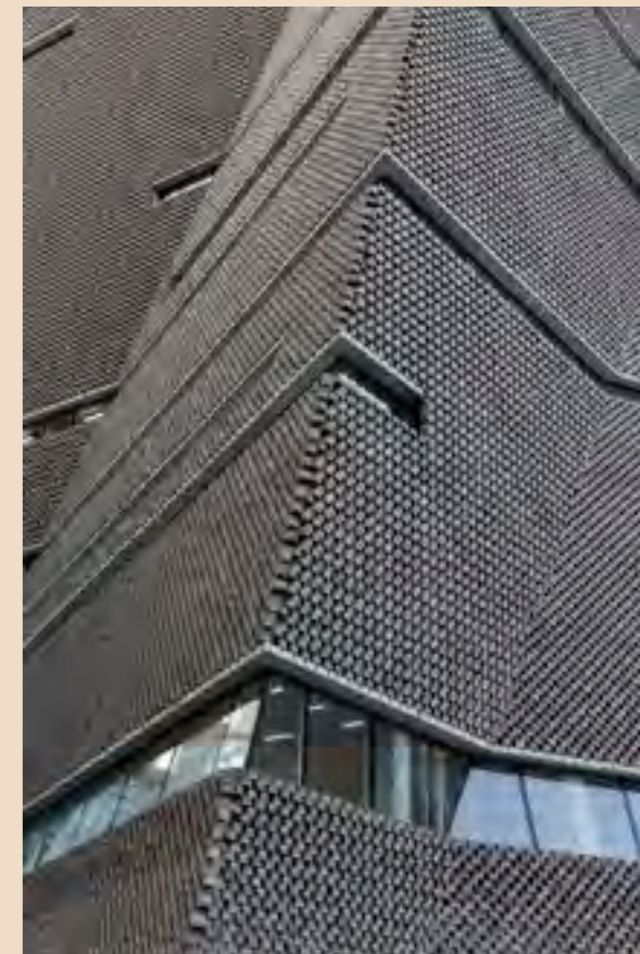
At Tate Modern, London, architects Herzog & de Meuron sought a modern brick to match that of the original building, a power station built in the 1940s.
