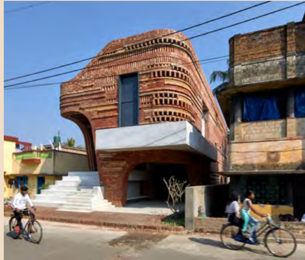
The unconventional shape of the building adds to the textural intrigue of Gallery House in West Bengal, India.
